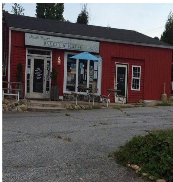
Courtesy of Greenville County
